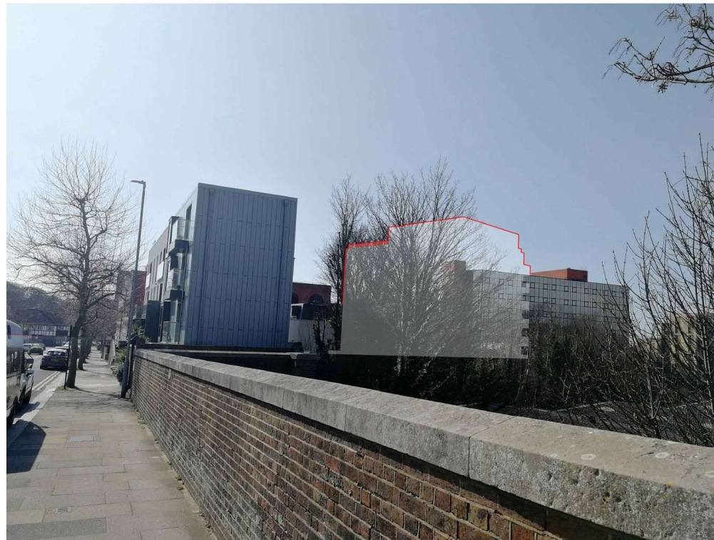
4 VIEW LOOKING SOUTH ALONG MONTEFIORE ROAD SCALE N/A
