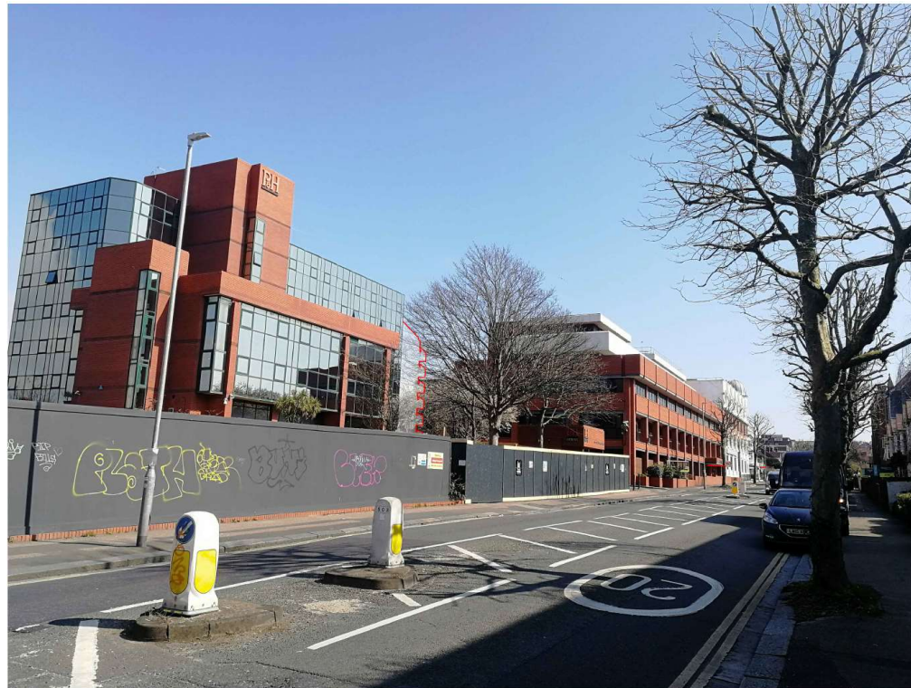
1 VIEW LOOKING EAST ALONG DAVIGDOR ROAD SCALE N/A
